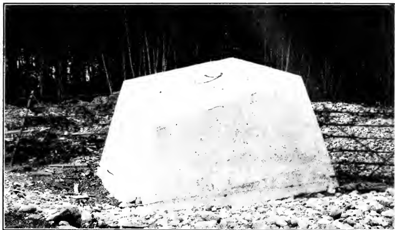
FIG. 8.—TYPICAL PIER, DRIFT BARRIER EXTENSION.
